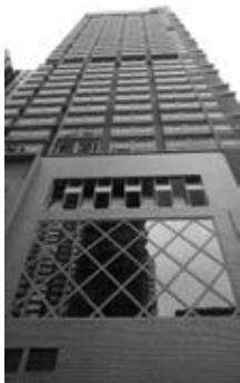
432 guest-room Best Western Hotel Harbour View Queen's Road West
