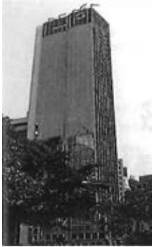
Shun Ho Tower Central
