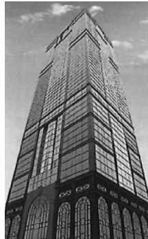
318 guest-room Ramada Hong Kong Hotel
